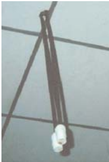
An improperly sized extension cord opens the door to arc or shock.
